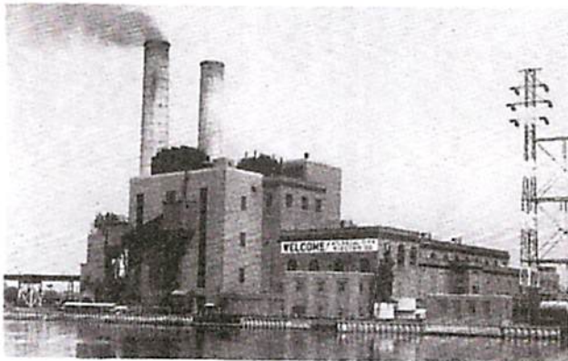
MISSOURI AVENUE GENERATING STATION CAPACITY 94,500 KW
