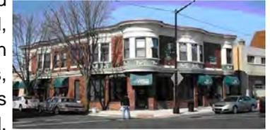
The second floor bay windows have Colonial Revival style decorative swags in the metal below the window openings. A pressed metal cornice (original) runs along the roof line and between the first and second stories.
