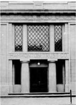
ca. 1915. Two-story Neo-Classical style bank is three bays wide and four bays deep. The façade (west elevation) features two, 1-story tall fluted columns placed in the recessed entrance; they support a three-part window (metal, modern) on the second floor. The center entrance is flanked by two tall windows; all appear to date to the mid-late 20<sup>th</sup> century. The Hammonton Trust Company was organized in 1908 at 104 Bellevue Avenue with A.J. Rider as president.
