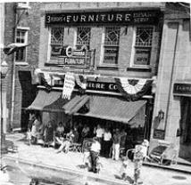
Ca. 1896-1903. It was built as a twin of the Hammonton Trust Company building. The painted metal cornice—one of the most decorative in town—has brackets, small rosettes, and half circle medallions and is capped on either end with large metal brackets, all original.
