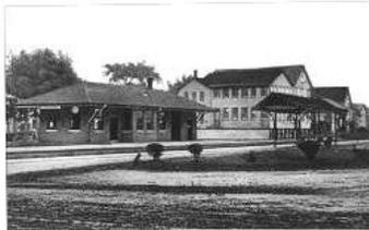
ca. 1904 – 1908. One story tan brick railway station. Shallow pitched, hipped roof extends to form a canopy that is supported by large knee braces (original).
