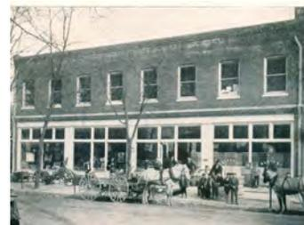
ca. 1900. Two-story, flat roofed, painted brick commercial building. The corrugated and diamond-patterned metal storefront of #124 is a well preserved example from a mid-20<sup>th</sup> century remodeling. The façade (west elevation) roof line features an original molded metal cornice with decorative modillions and crown molding.
